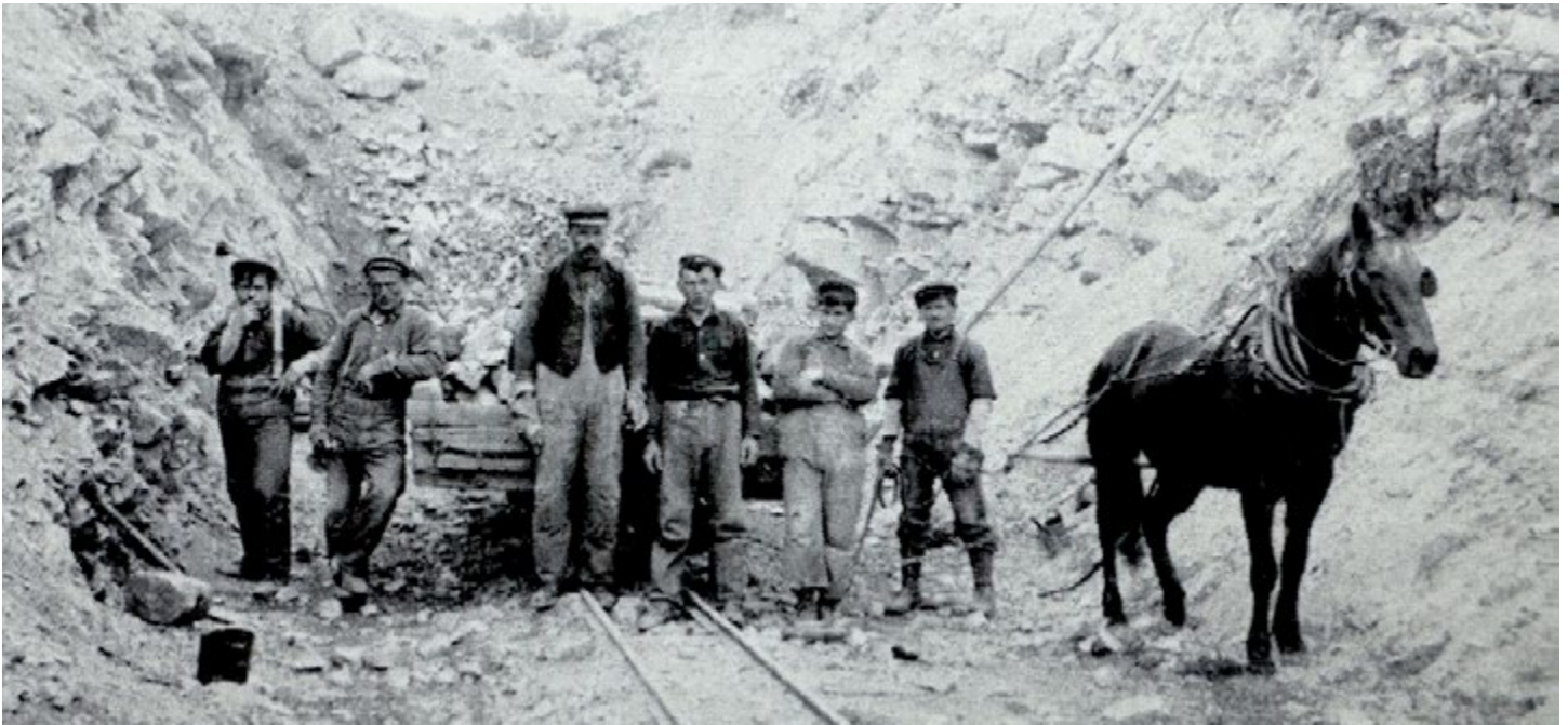
Workers clearing rock and debris from the railway right of way
