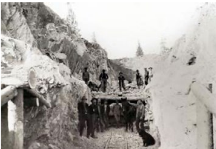
Working in a rock cut
