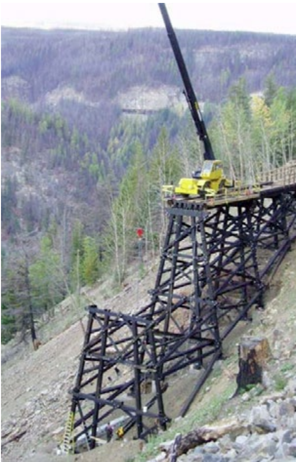
Rebuilding Trestle 11 after the fire
