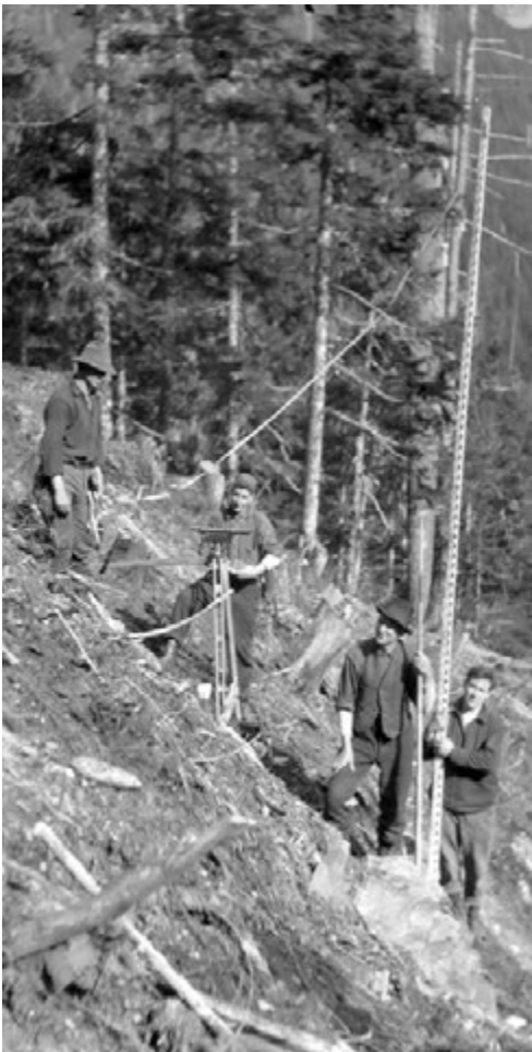
Surveyors at work laying the way
