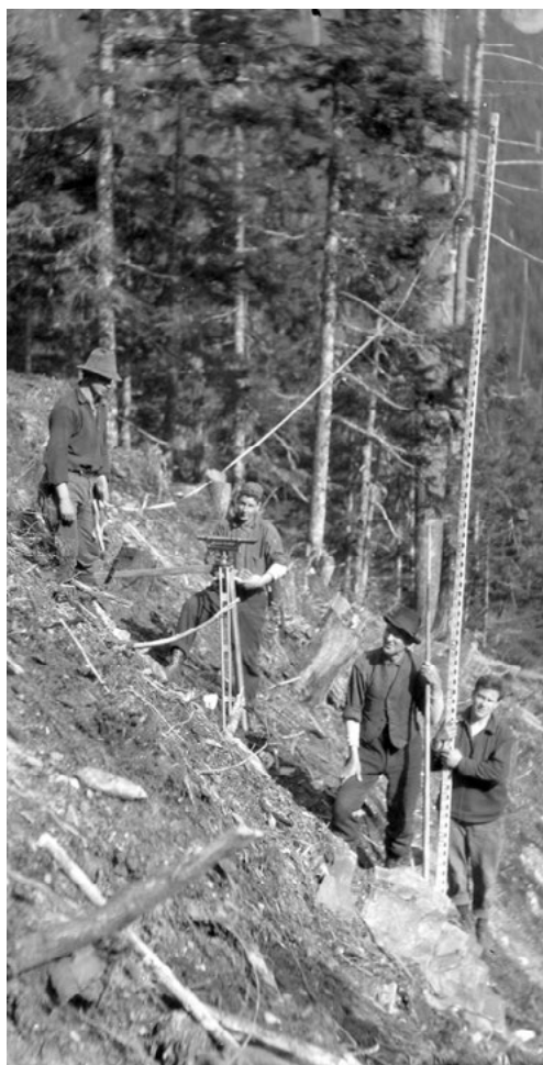
Surveyors at work laying the way
