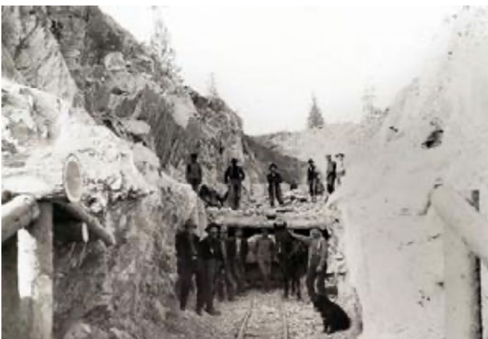
Working in a rock cut
