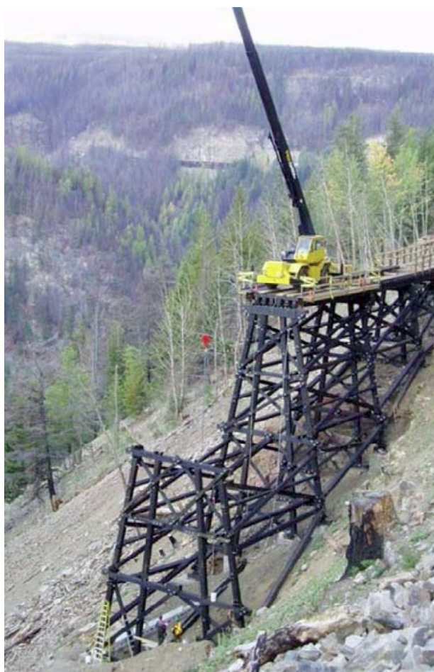
Rebuilding Trestle 11 after the fire
