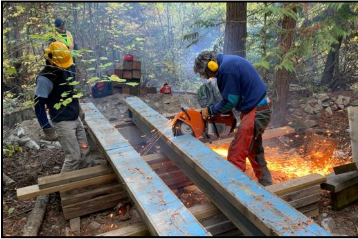
Constructing bridge supports on Fairlane Trail
