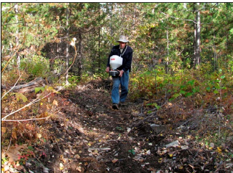
Gerry Gubbels seeding a drainage channel on Lost Lake Trail
