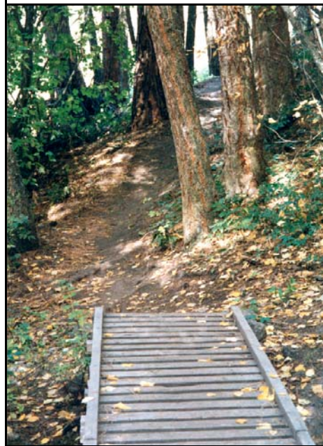
Bridge over Hachey Creek Oct. 02
